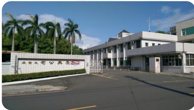
Taiwan – Kaohsiung Coating Research Center (1)
